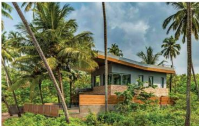
The concrete and tile material palette effectively discourages the build-up of moss on the walls of the structure, thereby enabling minimal maintenance (Studio IAAD)
