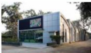
In order to reduce the heat gain, the west side has been blocked with a solid mass. Vertical strip windows were introduced on the west façade (Studio IAAD)
