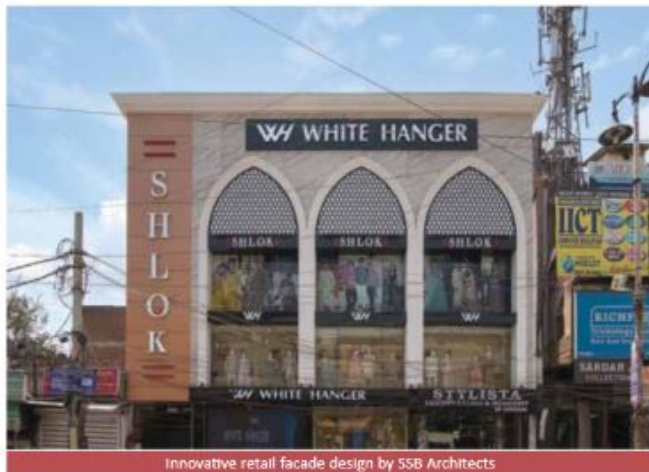
Innovative retail facade design by SSB Architects
