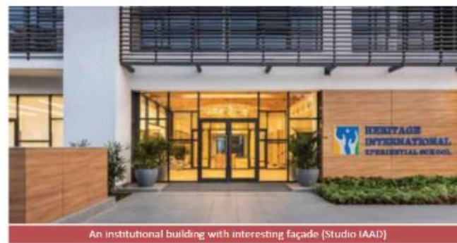
An institutional building with interesting façade (Studio IAAD)
